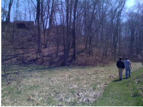
Figure 7: Trees growing vertically on top of the Lawyers Pt. landslide suggest that it is an older slide (Photo by Sarah Johnson).
