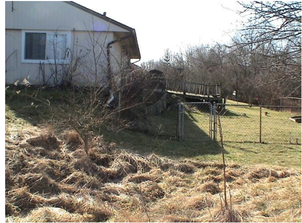
Figure 15: Photograph from 2005 of the backyard of one of the four homes directly affected by the large block extrusion failure at Huffman Ct. in Cincinnati, OH. The deck is shown slipping downwards away from the home indicating substantial movement (Photo by Sarah Johnson).
