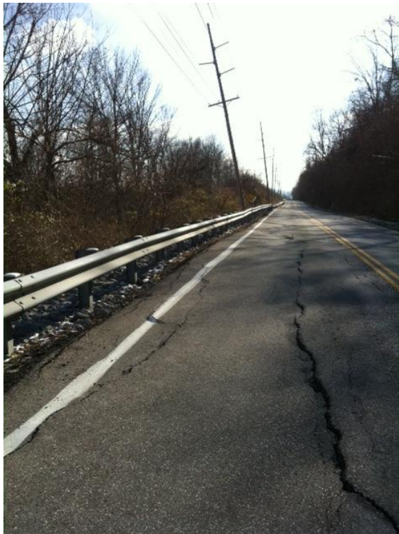
Figure 10: Many of the landslides on the steep slope on the south side of KY-8 have affected the road. These affects can be seen as cracks in the pavement, rolling or bumpy sections of road, and tilted utility poles (Photo by Sarah Johnson).
