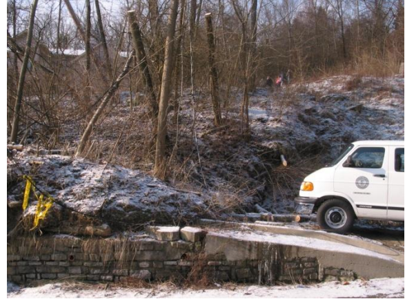
Figure 14: Photograph from 2005 of debris blocking the driveway off of Montague Rd. caused by a translational landslide. The slide was repaired after debris continually blocked the road (Photo by Sarah Johnson).
